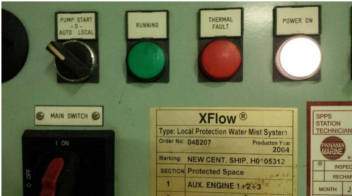
**Water Mist Control Panel in "Automatic" Mode with Electrical Power "On"**
