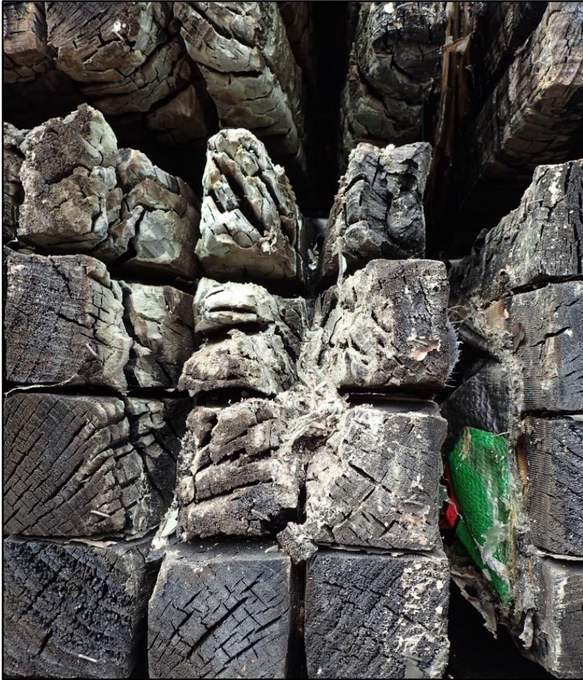
Figure 10 Charred timber at origin of fire
