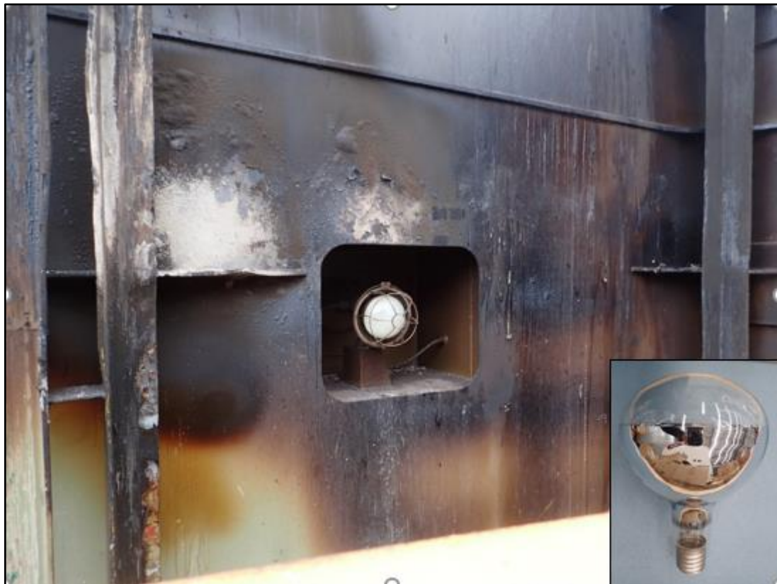
Figure 3 Cargo hold light in recess (inset, the reflector lamp)
